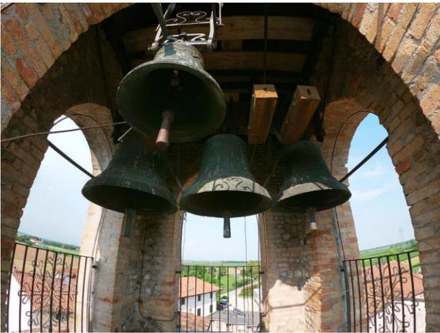
Figura 3. Example of belfry, Redenzicco (Udine). The bells of the main concert are manual (the only example of "string" bells in the territorial area) and jammed in the so-called "Friulian impulse" system. The support structure was made of metal.
