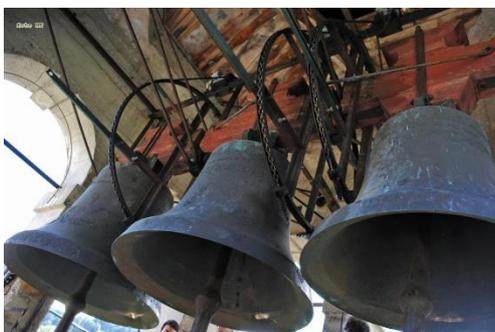
Figura 5. Example of "incastellatura" of bells in a structure with wooden blocks. The sound system in which the bells are mounted is the so-called "a slancio friulano".
