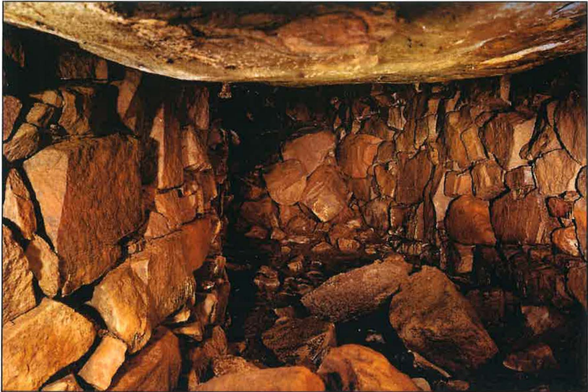
Medieval drystone souterrain inserted into the cairn of the Dowth Hall Passage Tomb.
