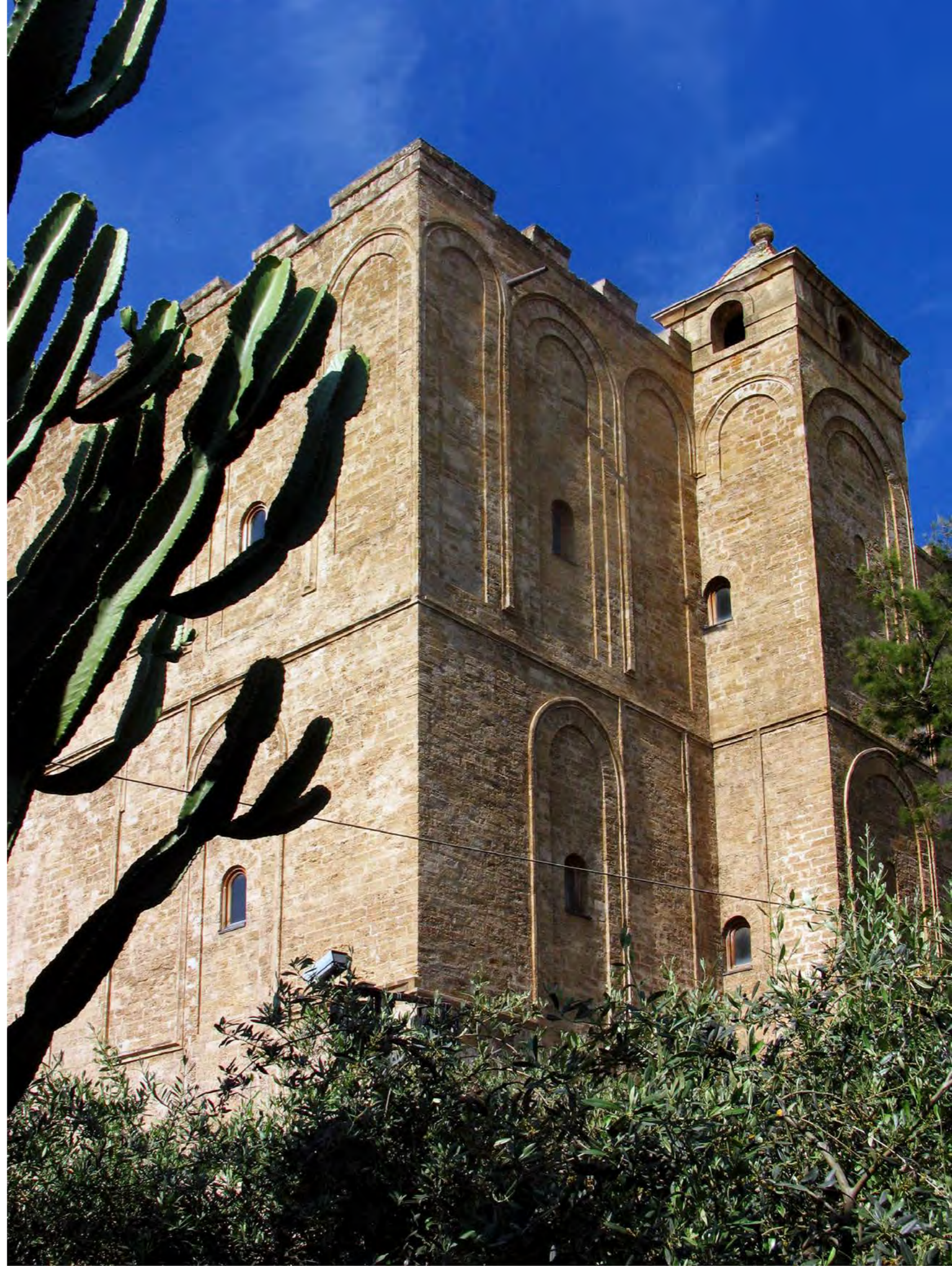
Zisa Palace, south-west corner.
