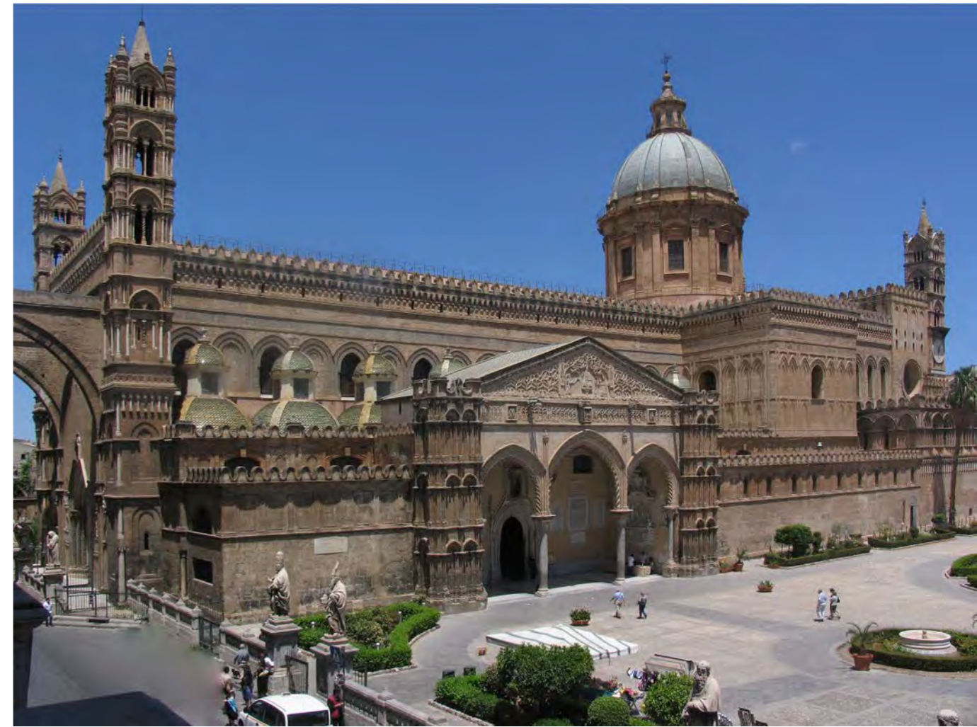
Palermo Cathedral, southern façade.
