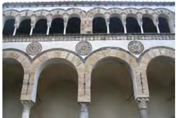
Fig. 5: Salerno, Cathedral of San Matteo, four-sided portico, detail with diachronic marquetries in lava stone, XII century. (source: web)
