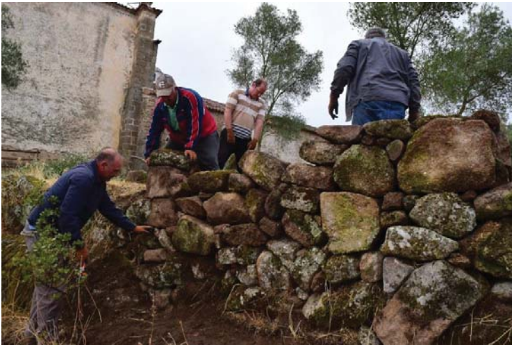
Bulding a dry Stone Wall ; Torrequemada, dehesa boyal
