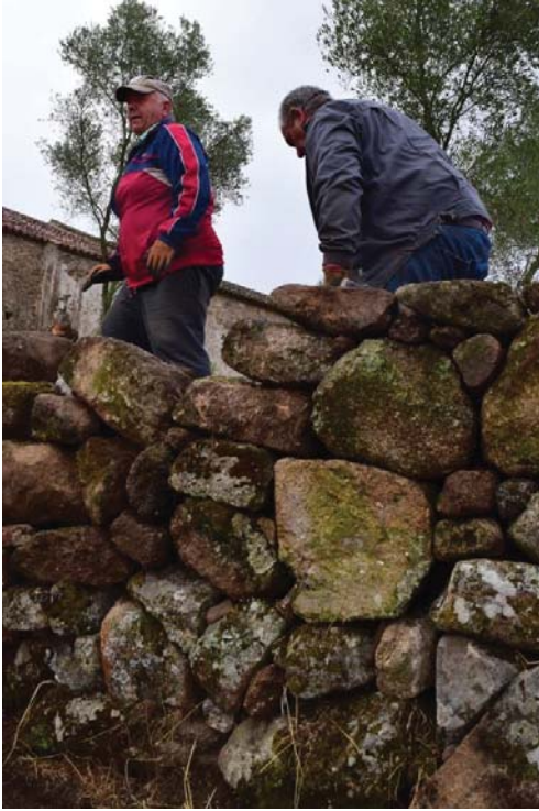
Bulding a dry Stone Wall ; Torrequemada, dehesa boyal III
