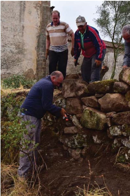
Bulding a dry Stone Wall ; Torrequemada, dehesa boyal
