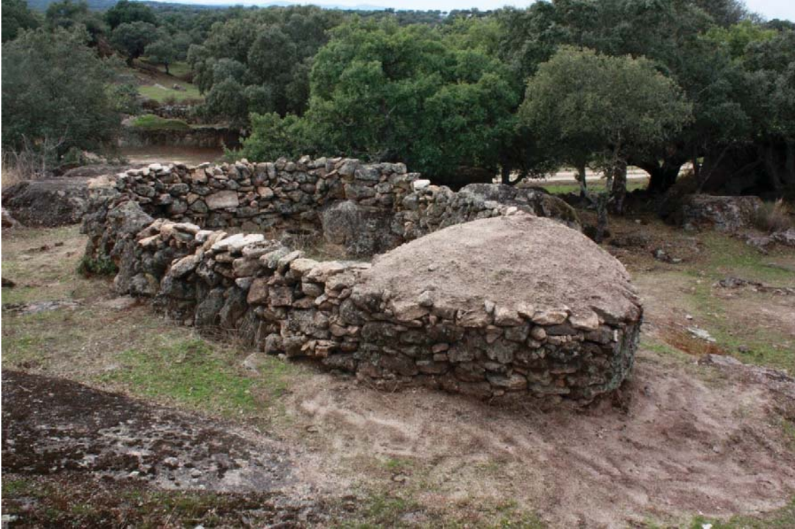
Restored Zahurda following the traditional technology of the stone dries
