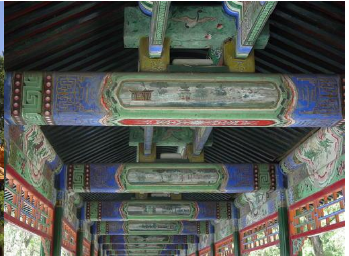
The Summer Palace after its renovation
